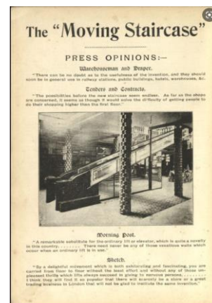
The First British Escalator
